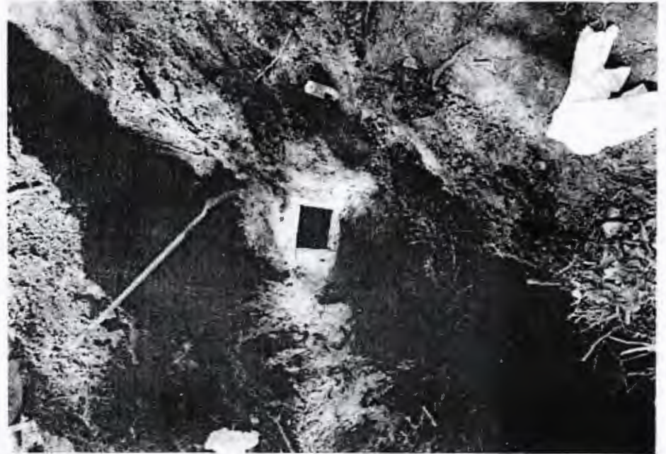
DURING INSTALLATION OF YARD DRAIN - 3/25/2021
